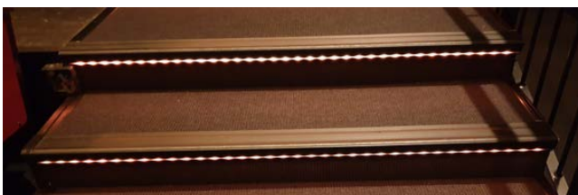
Stair light mounted in stair nosing, shining down along the risers.
